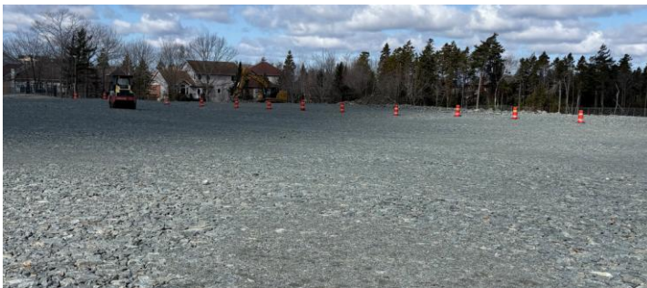
Grading and final elevation developed for south part of site
