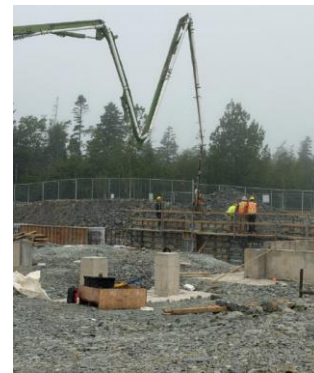
High foundation wall and retaining wall formwork installations Concrete pour for foundation walls and column piers
