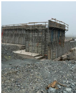
High foundation wall and retaining wall formwork installations Concrete pour for foundation walls and column piers
