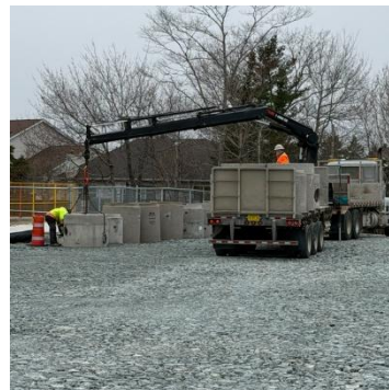
Delivery of catchbasins
