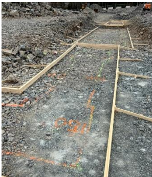
Formwork for footing mudslabs
