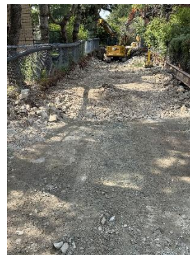
Sanitary and storm line installation ongoing
