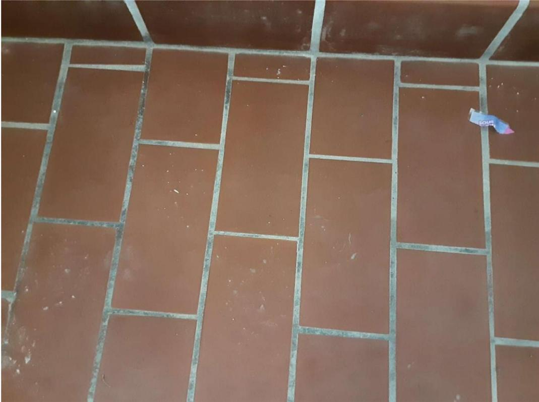
V9500 (Presumed Asbestos), Floor, Thin-set under ceramic tiles, Vestibule (Location #: 17)
