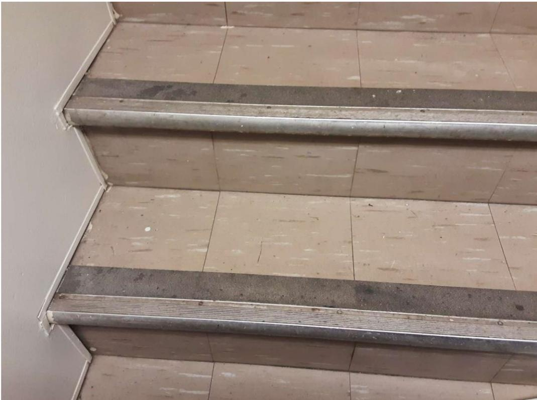
S0005A (Confirmed Asbestos), 9" tan, Floor, Stairs, Vinyl Floor Tile and Mastic, Landing and Stairwell (Location #: 6)
