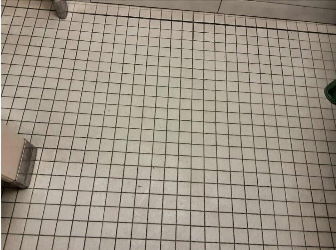
V9500 (Presumed Asbestos), Floor, Thin-set under ceramic tiles, Washroom (Location #: 11)
