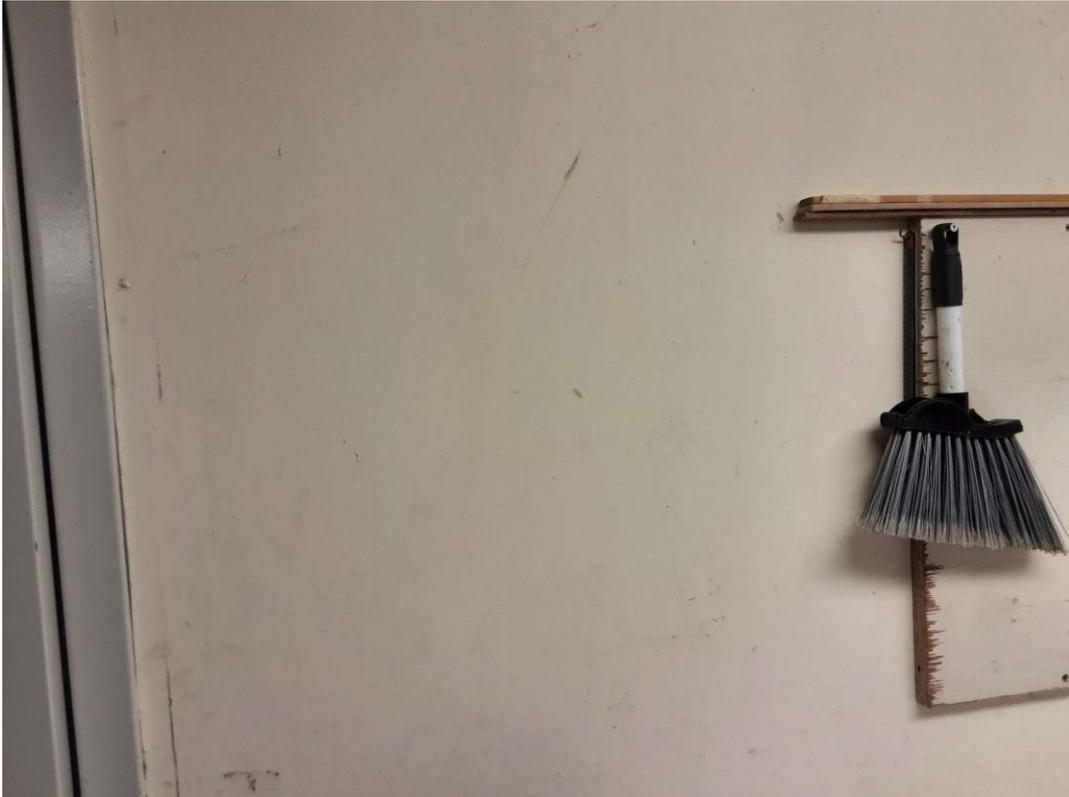
S0001A (Confirmed Asbestos), Wall, Drywall and joint compound, Old Boiler Room (Location #: 1)
