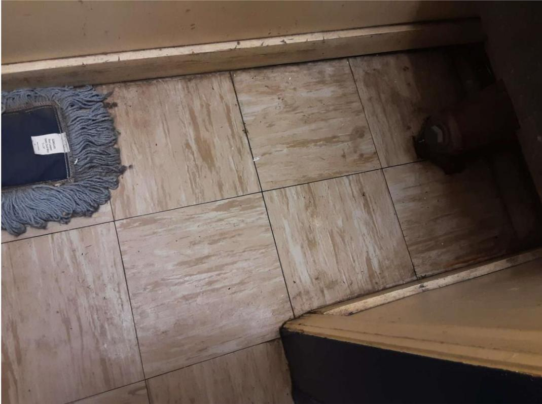
S0009A (Confirmed Asbestos), 12" beige with brown and white streaks, Floor, Vinyl Floor Tile and Mastic, Custodian Closet (Location #: 12)
