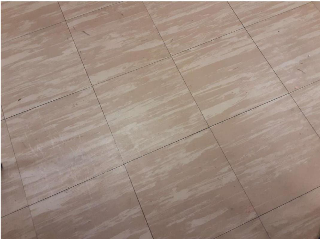
S0017A (Confirmed Asbestos), 12" beige with tan streak, Floor, Vinyl Floor Tile and Mastic, Classroom (Location #: 18)
