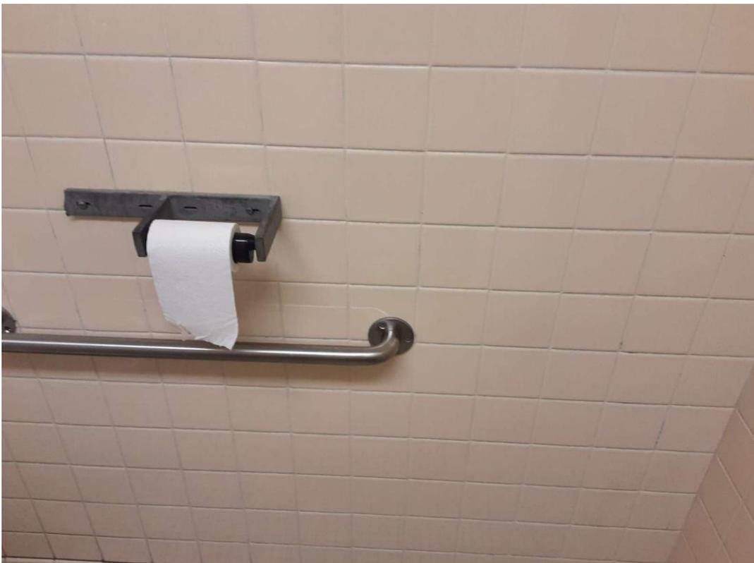
V9500 (Presumed Asbestos), Wall, Base, Thin-set under ceramic tiles, Washroom (Location #: 20)
