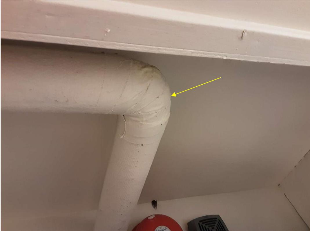
S0006A (Confirmed Asbestos), Piping, Parging Cement, Landing and Stairwell (Location #: 6)
