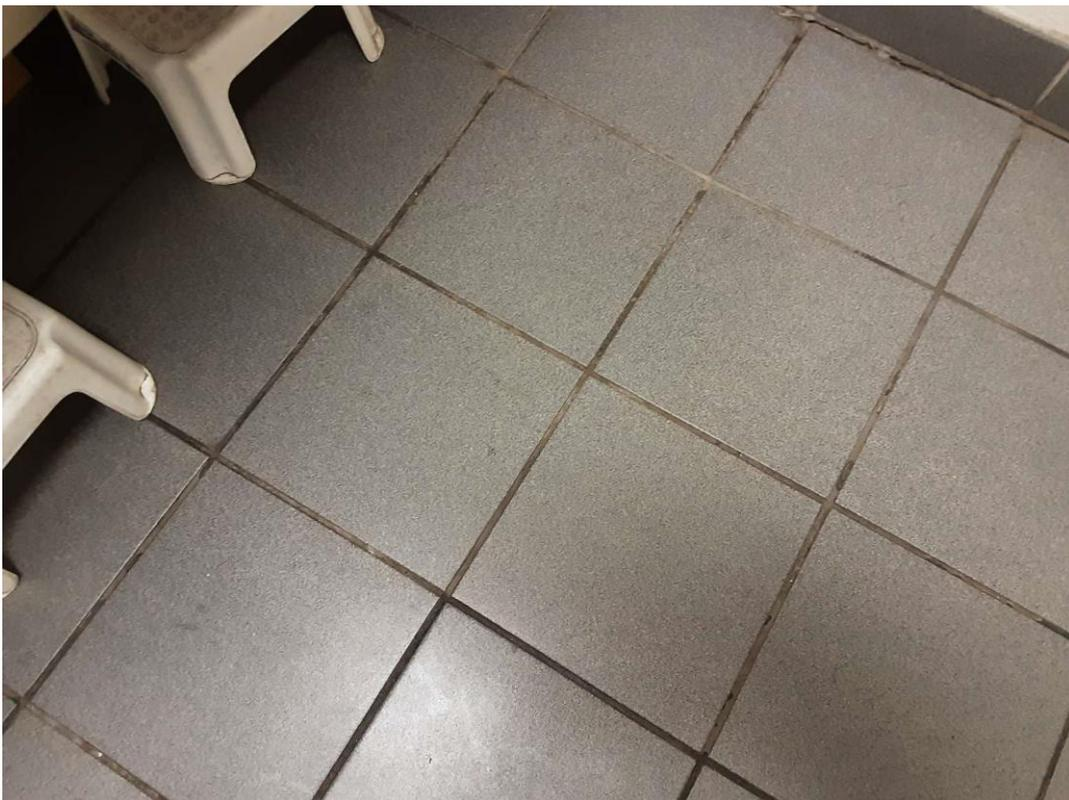
V9500 (Presumed Asbestos), Floor, Thin-set under ceramic tiles, Washroom (Location #: 13)
