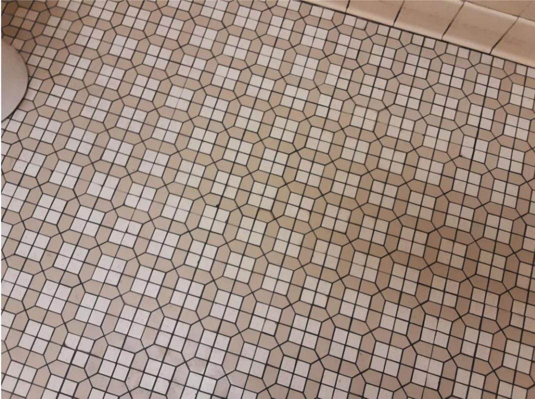
V9500 (Presumed Asbestos), Floor, Thin-set under ceramic tiles, Washroom (Location #: 20)
