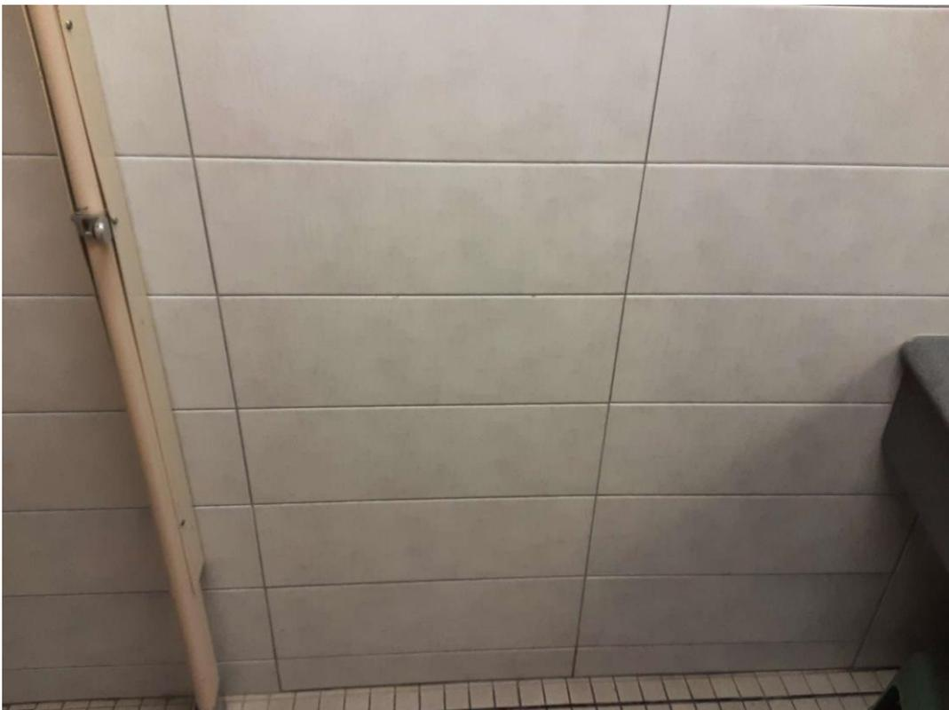
V9500 (Presumed Asbestos), Wall, Base, Thin-set under ceramic tiles, Washroom (Location #: 11)
