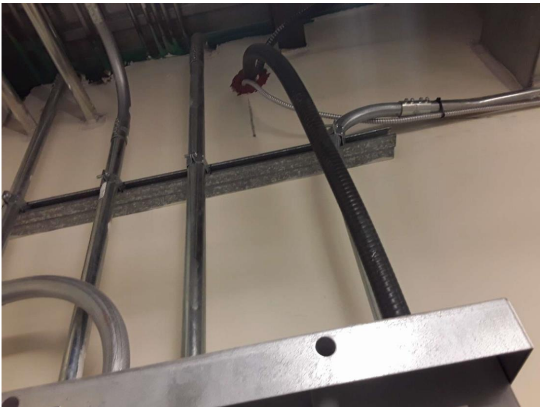
S0002A (None), Red fireproofing mastic on electrical conduit, 1F Electrical, General Storage, Custodial (Location #: 8)
