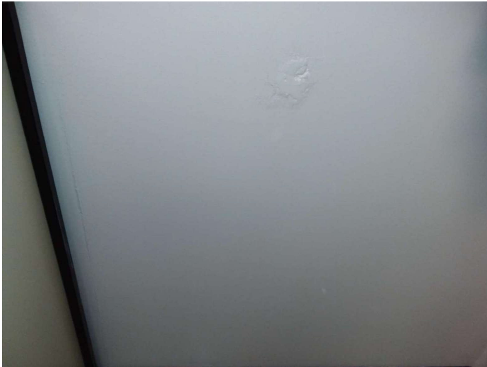
Lead, Low (L0007) Wall, Office (Location #: 30) Grey
