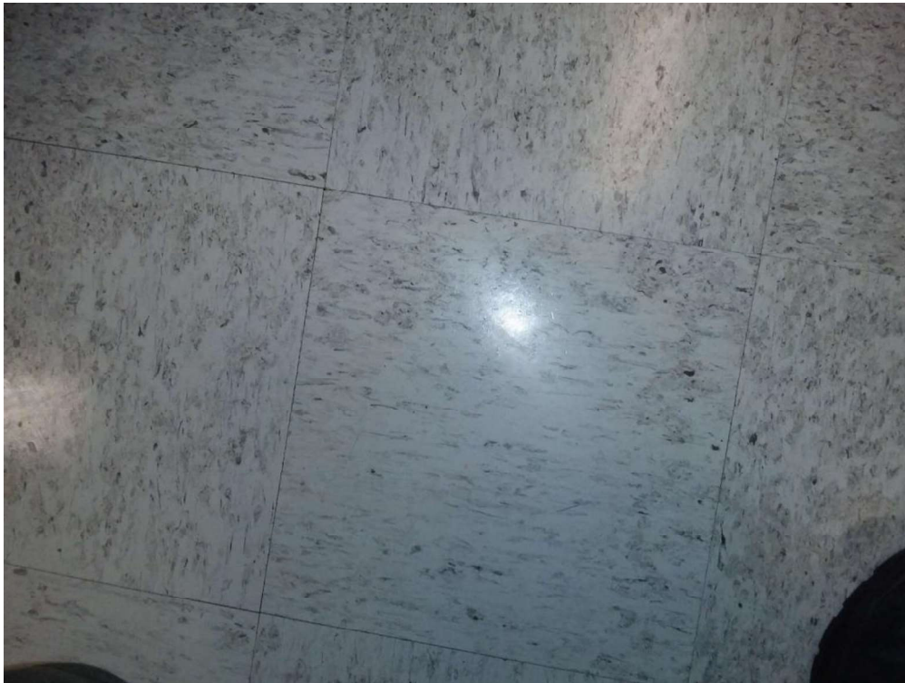
Confirmed Asbestos (detected in the tile, S0007A-C), 12" grey with black patterns, Floor, Vinyl Floor Tile and Mastic, Classroom (Location #: 2)
