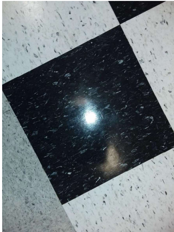
Confirmed Asbestos (detected in mastic, S0018A-C) 12" black with white streaks, Floor, Vinyl Floor Tile and Mastic, Resource Room (Location #: 18)
