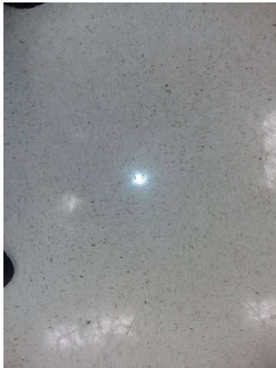
Confirmed Asbestos , detected in the tile, mastic is presumed, S0010) 12" light green with dark flecks, Floor, Vinyl Floor Tile and Mastic, Classroom (Location #: 4)
