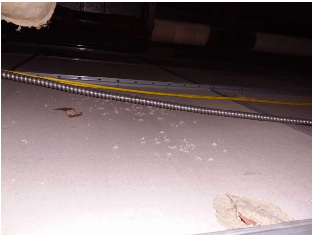
Confirmed Asbestos (S0011A-C), Piping, Debris, Parging Cement, Sewing Lab (Location #: 14)
