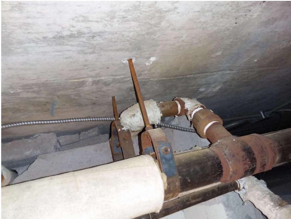
Confirmed Asbestos (S0011A-C) Piping, Parging Cement, Sciences Lab Storage (Location #: 12)
