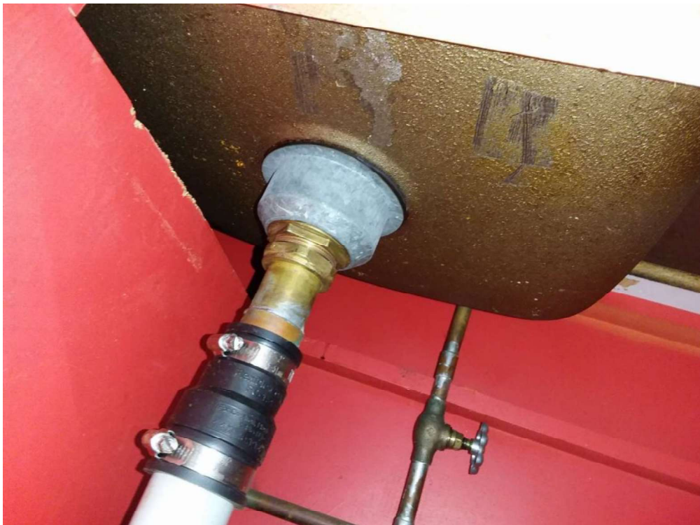
Confirmed Asbestos (S0017A-C), Gold Sink Mastic, Sewing Lab (Location #: 14)
