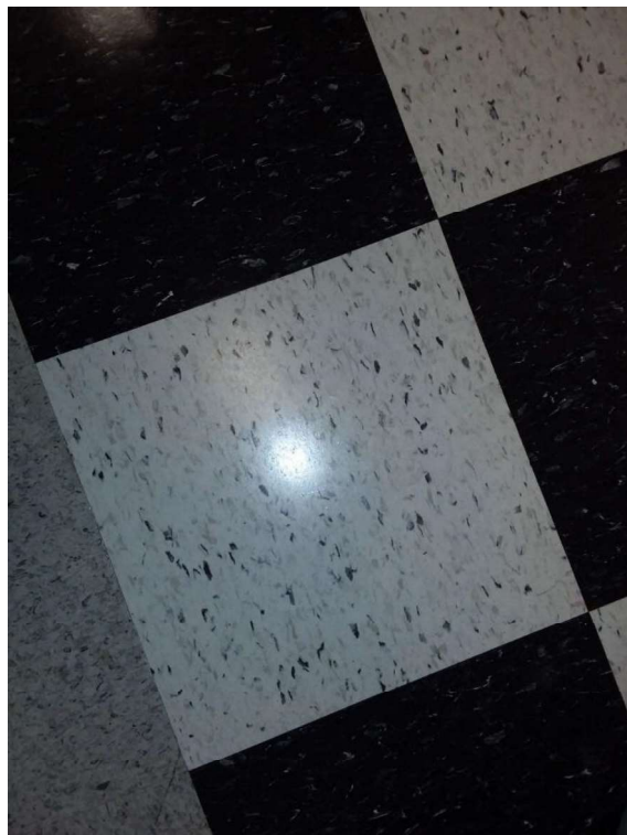
Confirmed Asbestos (detected in mastic, S0019A-C), 12" white with black streaks, Floor, Vinyl Floor Tile and Mastic, Resource Room (Location #: 18)
