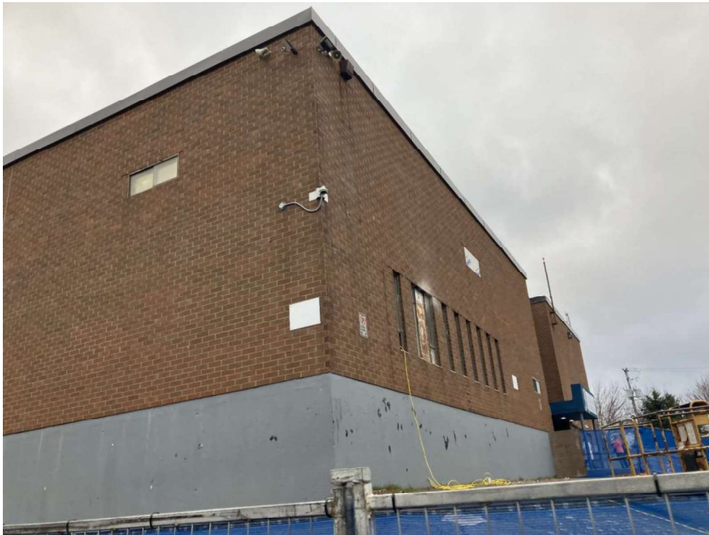
Lead, None (L0011) Wall, Exterior (Location #: 75) Blue
