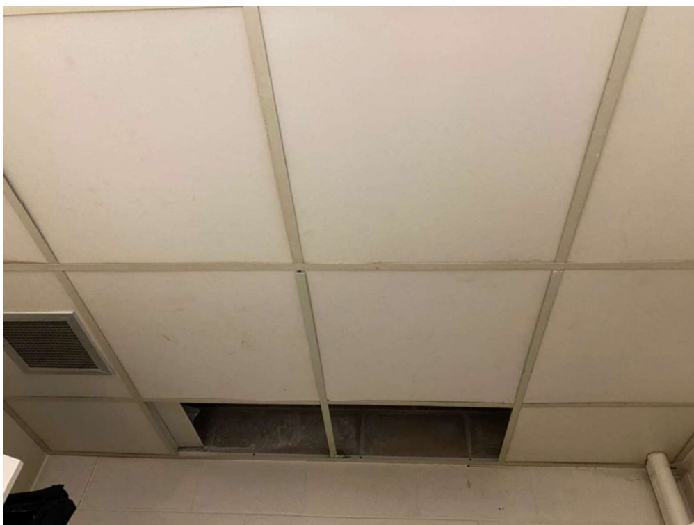
Confirmed Asbestos (V9000), 2x2 Transite, Ceiling, Cement Product, Storage Room (Location #: 76)
