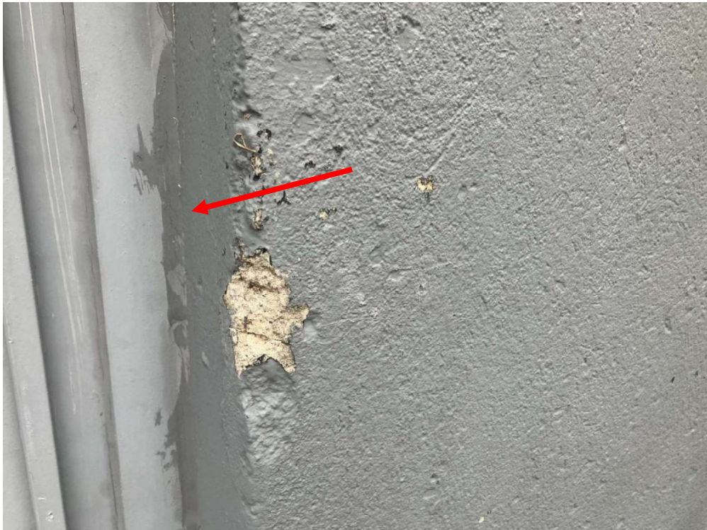
Confirmed Asbestos (S0026A-C), dark grey, Wall, Caulking, Exterior (Location #: 75) between exterior window and wall
