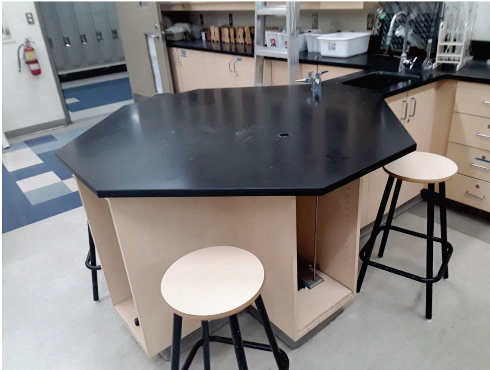
V9500 (Presumed Asbestos), Other, Bakelite countertops, Chemistry Labs (Section A) (Location #: 43) Laboratory bench tops
