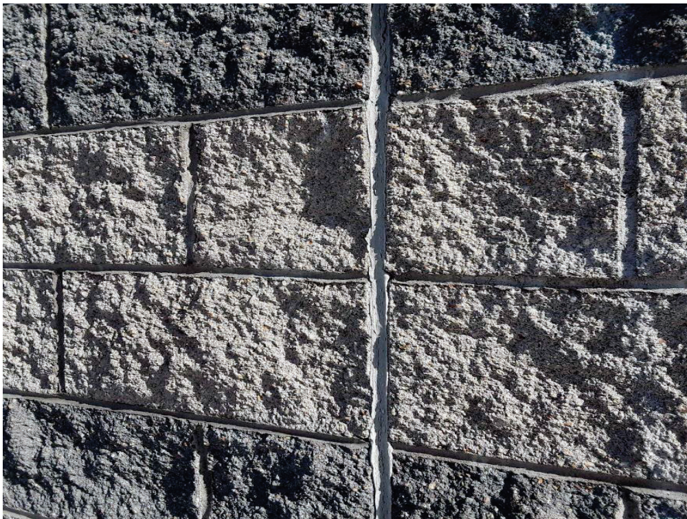
S0005A (None), Expansion Joint, Caulking, Grey, Exterior (Location #: 46)
